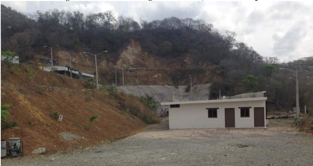
Figure 18.2 View of Existing Infrastructure, San Rafael Project
