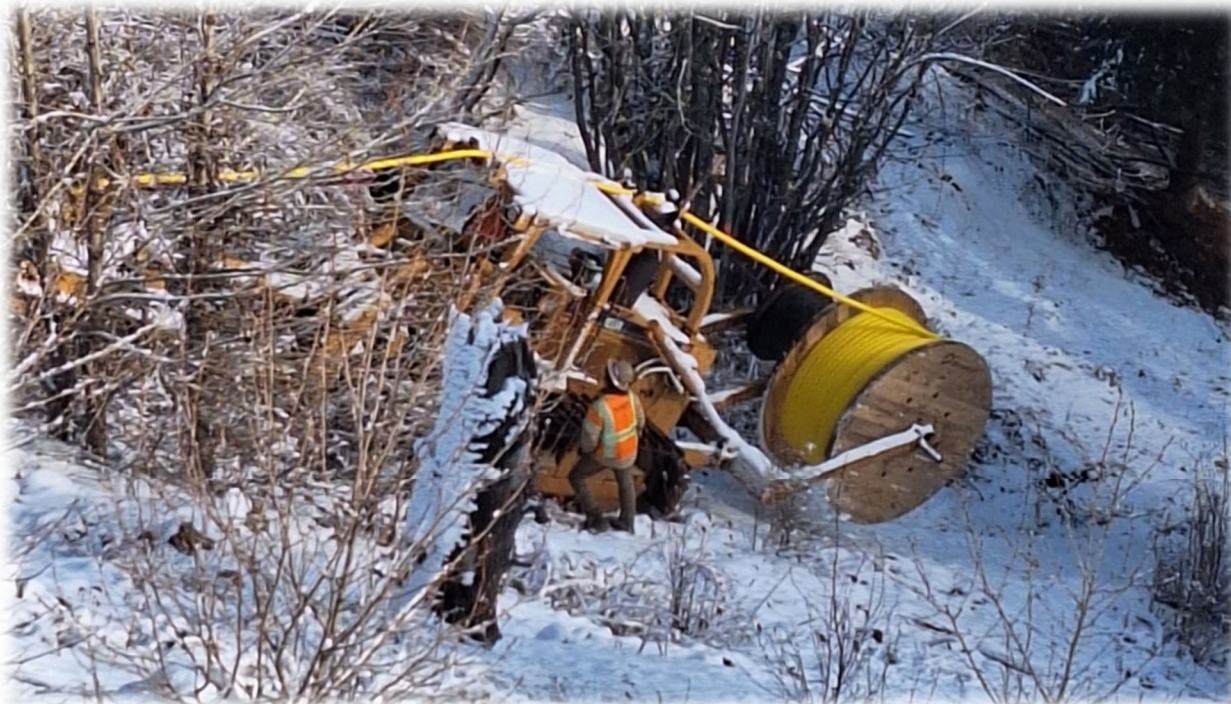
Figure 1: Connecting grid power to the hooper adit – ripping a cable trench using a D-6 CAT Cable Trencher
