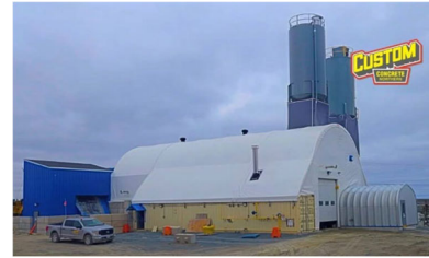
Custom Concrete Mixing Plant
